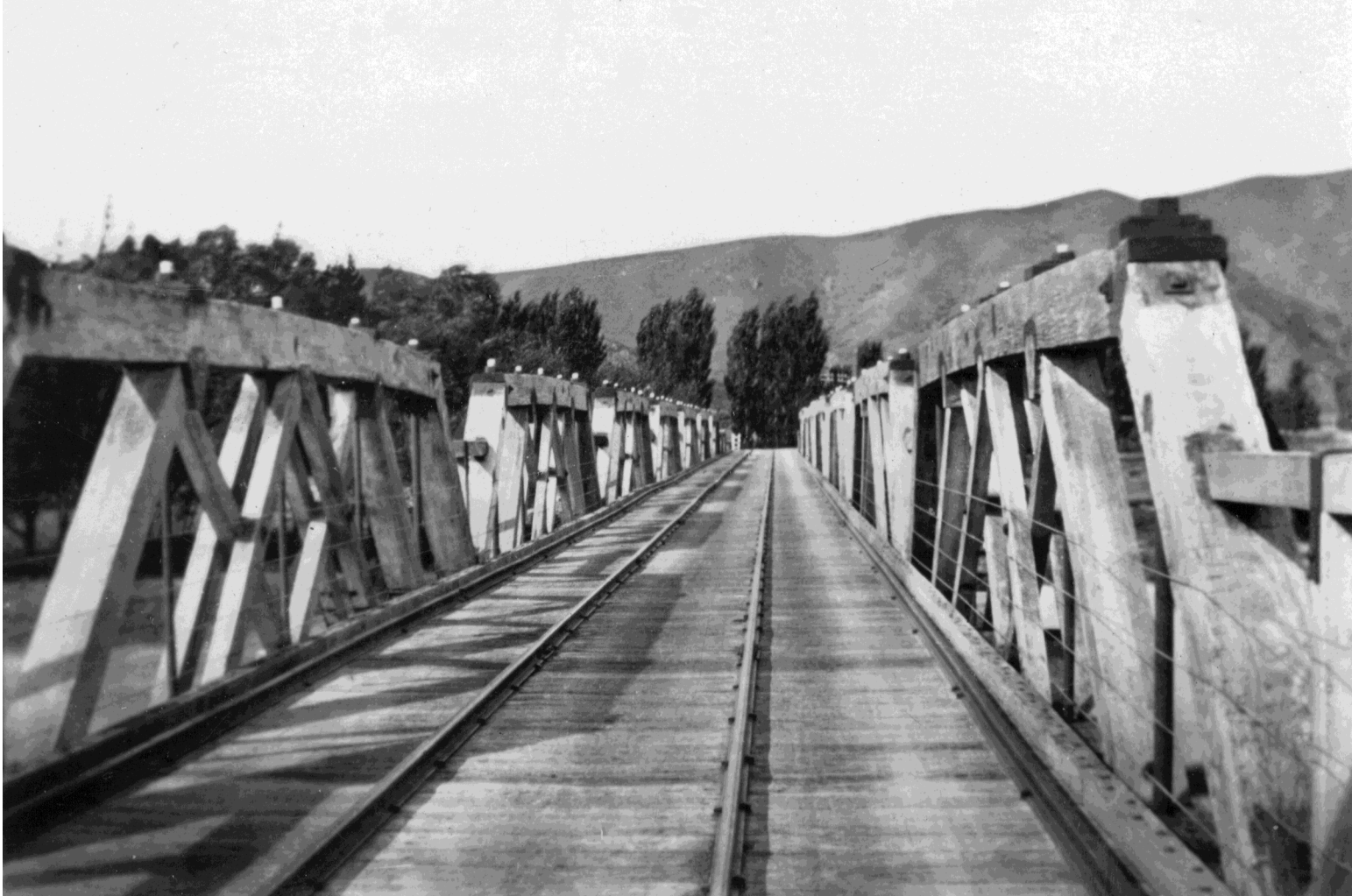
WAITAKI ROAD RAIL BRIDGE
